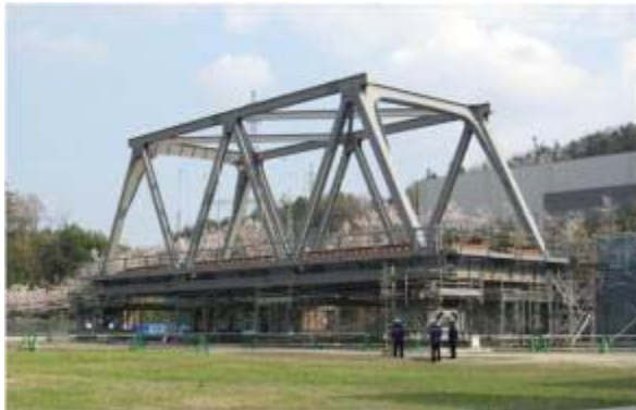
Truss Bridge (for tests)
