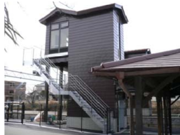
Installation of Elevator at a station (Kamezaki Station)
