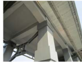
Large-scale Renovation (Concrete Viaduct: measures to inhibit age-related deterioration)
