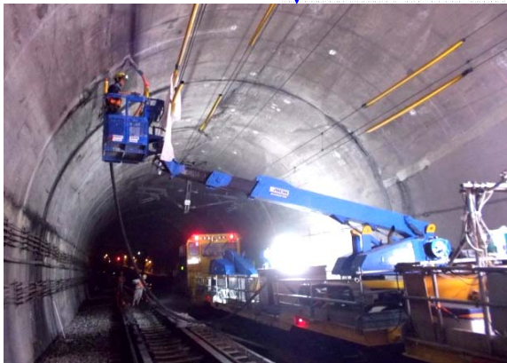
Example of the Large Scale Renovation (Tunnel)
