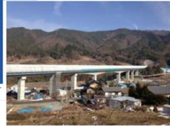
Bridge (over a river)
