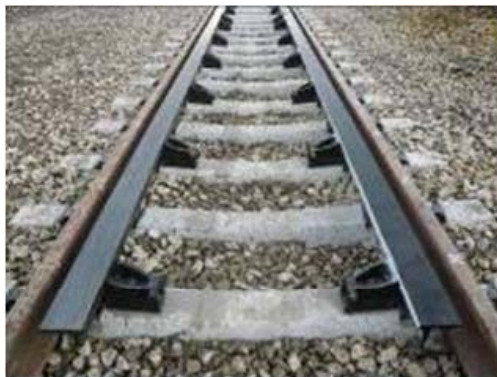
Countermeasures for Derailment and Deviation (Tokaido Shinkansen)
