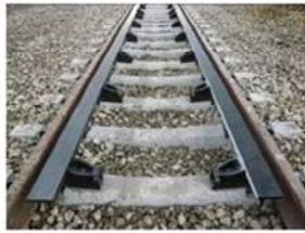
Countermeasures for Derailment and Deviation (Tokaido Shinkansen)
