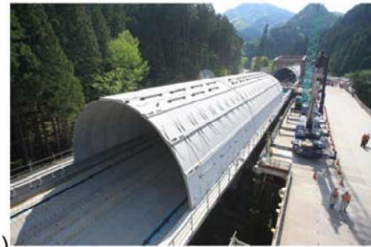
Yamanashi Maglev Test Line Construction Site at the Akiyama region, Uenohara City
