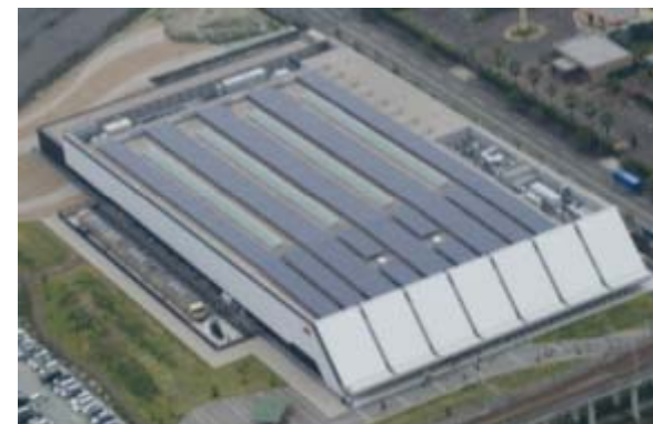
Photovoltaic Power Generation System (SCMAGLEV and Railway Park)
