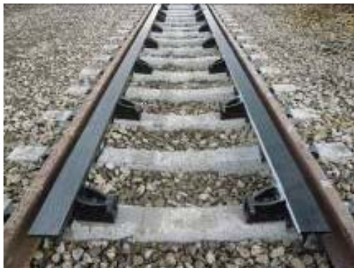
Countermeasure for Derailment and Deviation of the Tokaido Shinkansen
