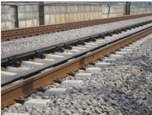
Countermeasure against Derailment and Post Derailment of the Tokaido Shinkansen
