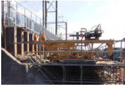
Quake-resistant Reinforcement of Embankments of the Tokaido Shinkansen
