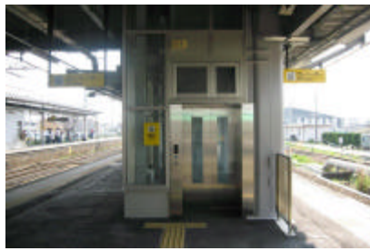
Installation of Elevators
