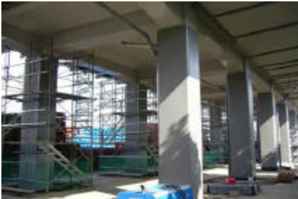
Quake-Resistant Reinforcement of Elevated Track Columns of the Tokaido Shinkansen
