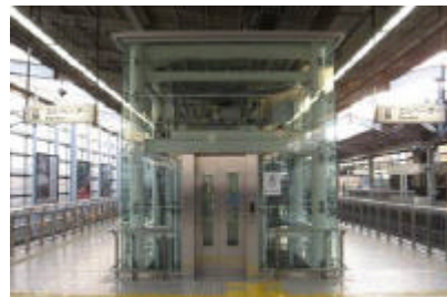
Installation of Elevator
