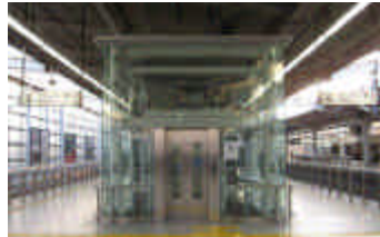
Installation of Elevator
