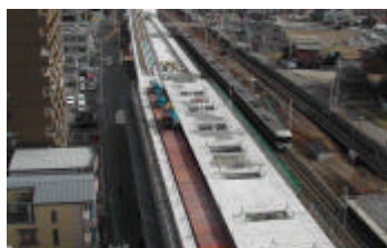
Elevation of railway track (Kachigawa)
