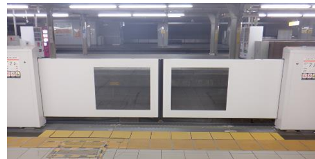
Concept image of movable platform fences to be installed on Platform 2 at Nagoya Station (The photo shows the movable platform fences already installed on Platform 5.)
