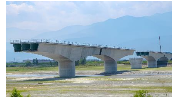
Superstructure of Kamanashi River Bridge
