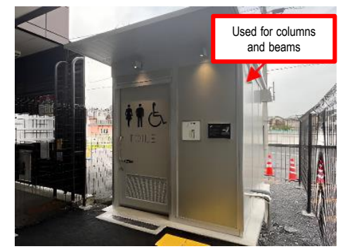
Examples of the use of recycled aluminum from the Tokaido Shinkansen (Building materials used in the restroom at Tobu Railway's Kuzu Station)
