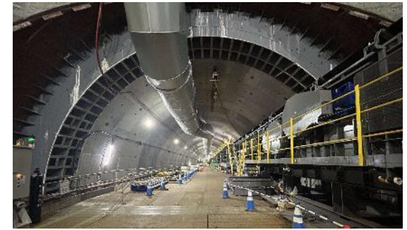
Chukyo Area Tunnel No. 1 (Meijo Section) Full-scale excavation
