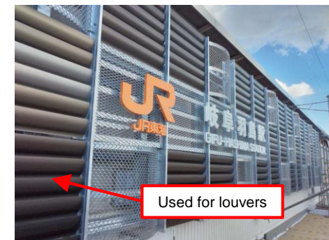
Examples of the use of recycled aluminum from the Tokaido Shinkansen (Used as a building material for condominiums and for the exterior of Gifu-Hashima Station on the Tokaido Shinkansen line)
