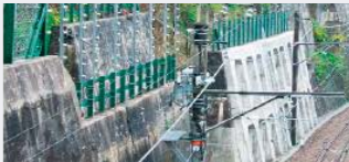
Falling rock retaining walls and alarm devices
