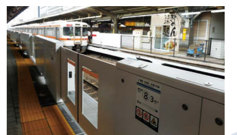
Movable platform fence on Platform 7 at Nagoya Station
