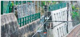
Falling rock retaining walls and alarm devices
