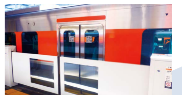
Platform fences on Platform 6 of Nagoya Station
