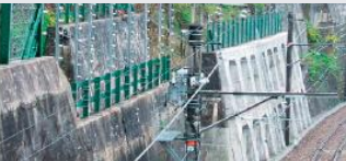
Falling rock retaining walls and alarm devices
