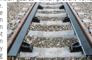
Derailment prevention guards
