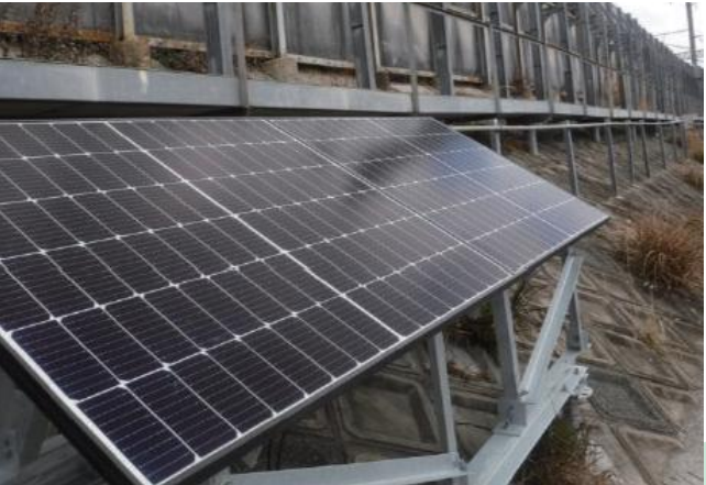
Solar power generation using the Shinkansen trackside slope (trial installation)
