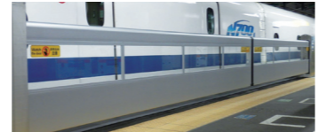
Platform fences on Platform 20 of Shin-Osaka Station
