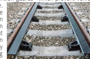
Derailment prevention guards
