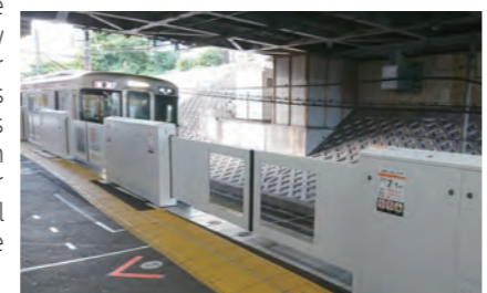
Installation of platform fences on Platform 4 of Kanayama Station
