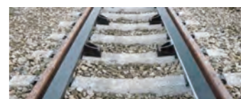
Derailment prevention guards
