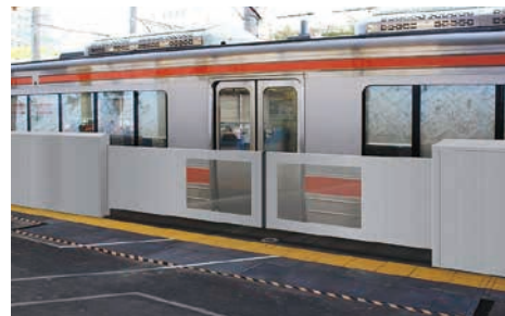
Image of movable fence (The photo shows a prototype fence at Kanayama Station.)
