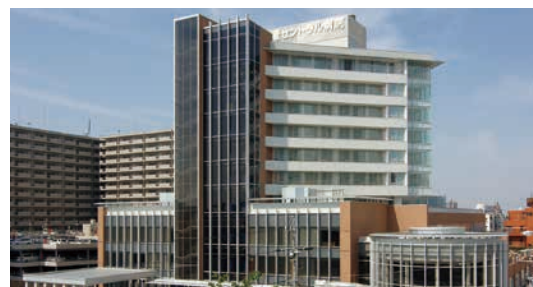
Nagoya Central Hospital
