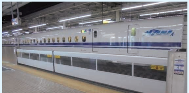
Large-opening movable platform fence at Shin-Osaka Station Platform No. 26
