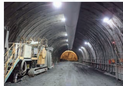
Southern Alps Tunnel (Yamanashi construction area)
