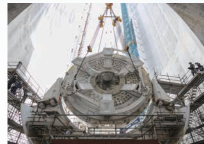
Shield machine assembly (North Shinagawa Emergency Access)
