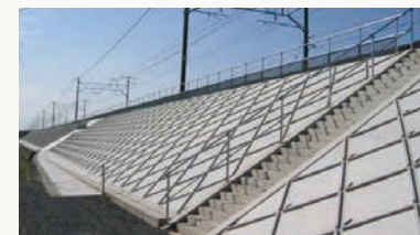
Slope protection work
