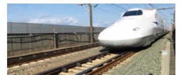
Derailment prevention guards
